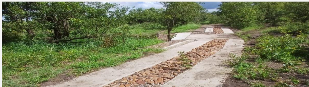
Figure 7.26: Safe crossing over a wetland/watercourse in the Kruger National Park – This structure aids game rangers with safe and quick access to sites over watercourses to fight against poachers. The structure ensures that the vehicles do not disturb the wetland soils, protects the wetland from erosion and allows for free flow of the watercourse over the structure (Source: DFFE)
